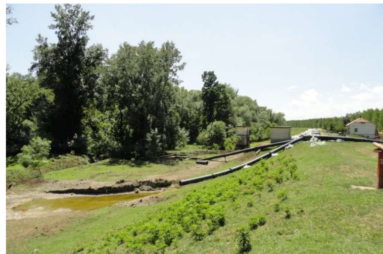
Figure 54: Pumping station Lipac near Jamena. Additional pipes over dike after the flood in 2014. (Source: ALEN KIS).
